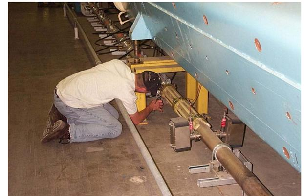
Air-core quadrupole being installed at E0. The magnets clamp onto the existing beam pipe without any need for breaking vacuum.
