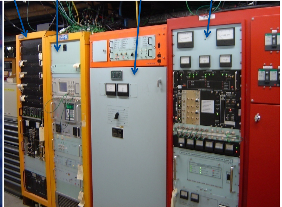
Upgraded RF Station with SSD + New Modulator
